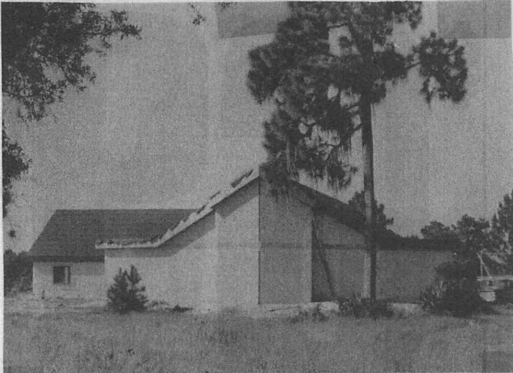
Building progress continues on Spring Lake Presbyterian
