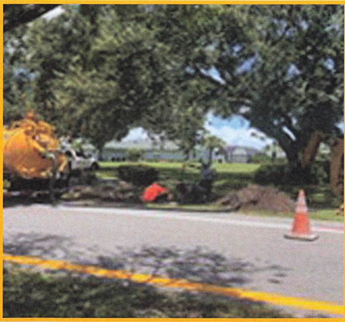
District Staff promptly respond to water leaks and breaks.
