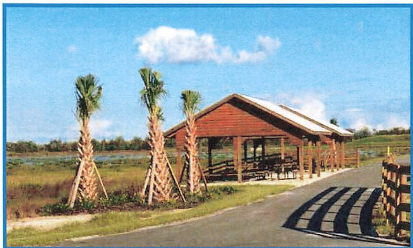
The Storm Water Treatment Project (ECO Park) broke ground October 31, 2014
